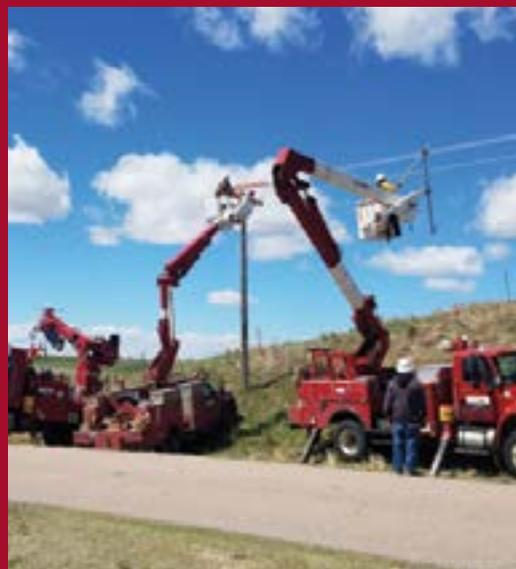
Linemen for High West Energy replacing a utility pole to ensure reliable electric system to our members.
